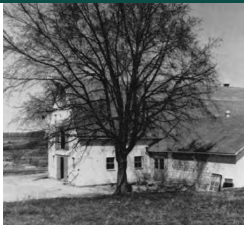
Beginning in the fall of 1963 the "Barn" was converted into a gymnasium.
