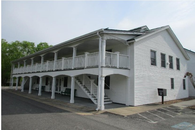
B10 - Multi-Story - Wood Frame - 1934
