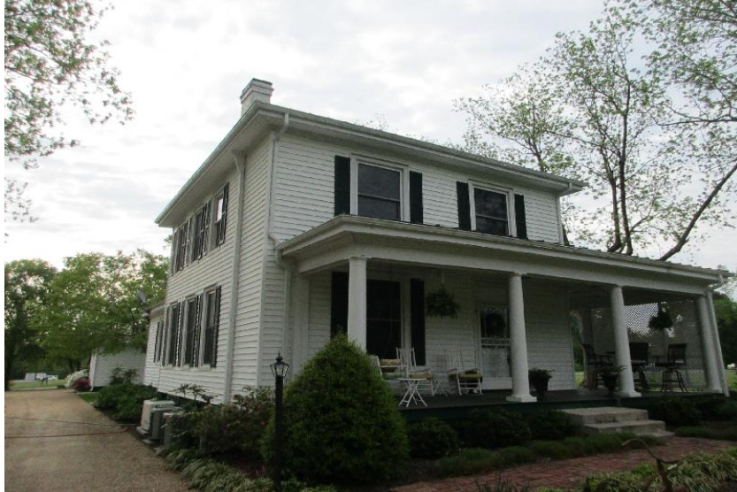
B10 - Multi-Story - Wood Frame
