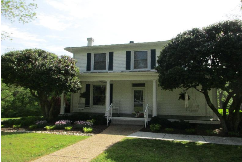
B10 - Multi-Story - Wood Frame - 1925
