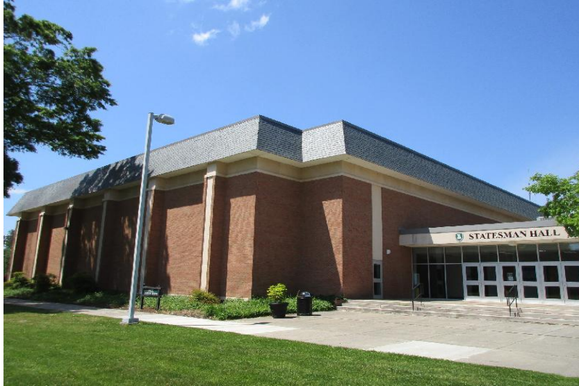
B10 - High Bay - Steel Frame with Composite Steel Roof Deck - Gymnasium Court
